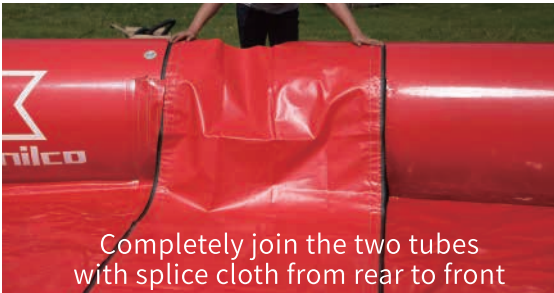
Join the tubes after fully inflated
