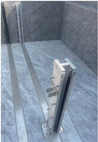
304 stainless steel base plate under aluminum flood barrier.
