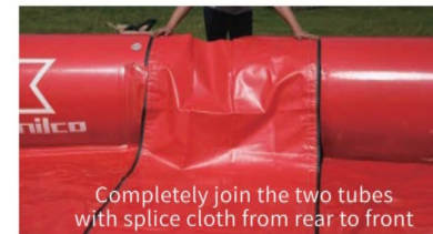
Adjoin the tubes after fully inflated
